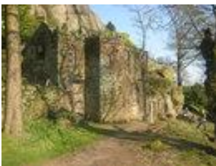
A closer view of Rock Hall Cottage
