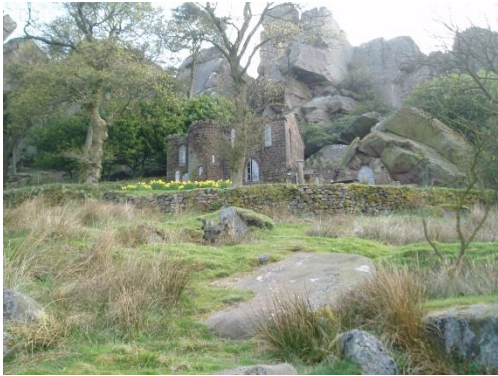
Rock Hall Cottage
