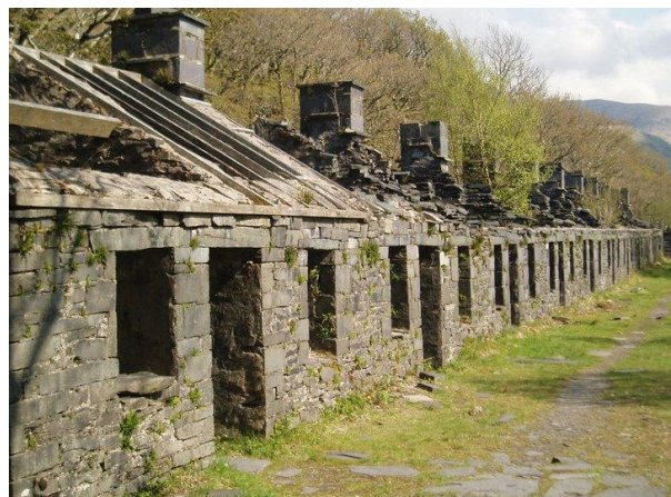
Anglesey Barracks, where the workmen lived 6 days out of 7, Sunday they could go home to Chapel
